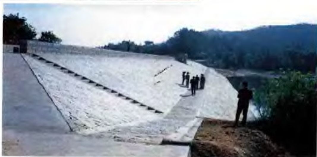
加固后之石獅灵 秀山水库大坝 ▶
