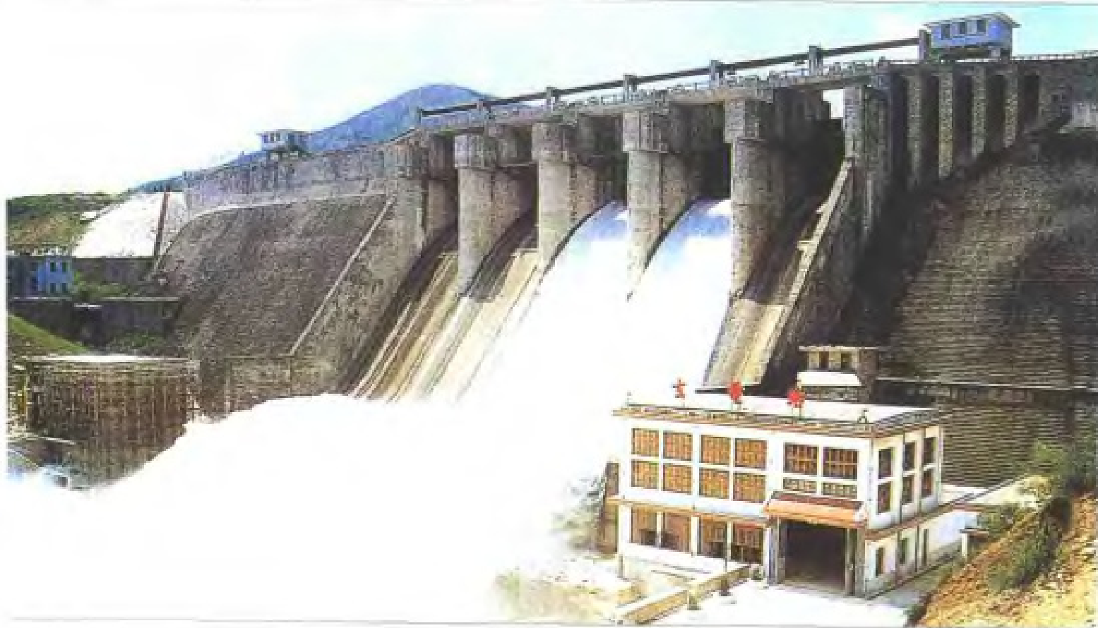
峰头水库大坝
